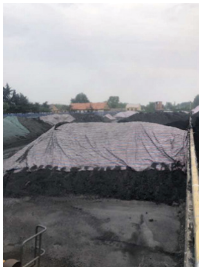
Preparation work for the expansion of Eastern Platform
