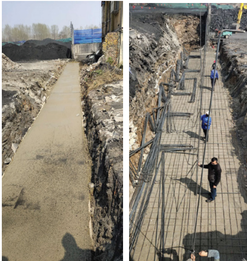
Cement and Concrete were used to reinforce steel to strengthen and widen the cargo platform at Shandong Kailai
