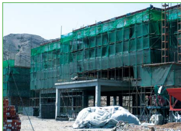
Construction of Office Building
