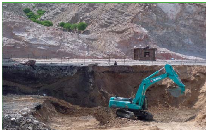
Construction of Boiler Room
