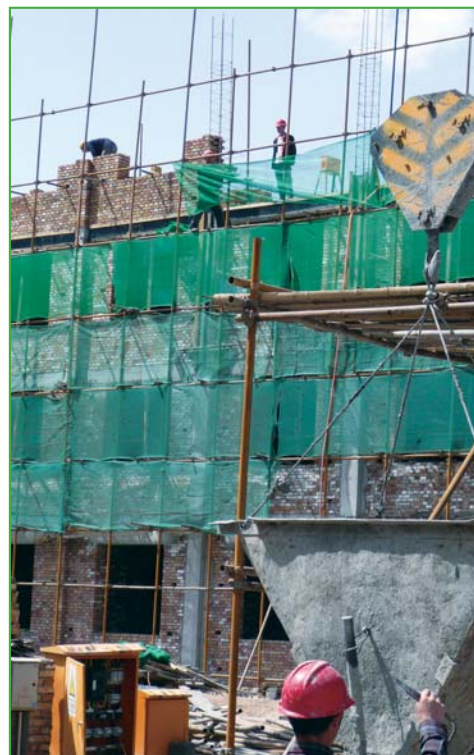
Construction of Staffs Quarter
